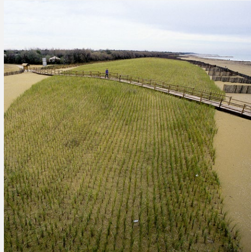
12 km Dune Restoration
