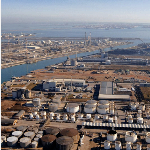
40 km Industrial Channel banks insulated and waterproofed
