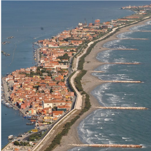
56 km Protected beach nourishment
