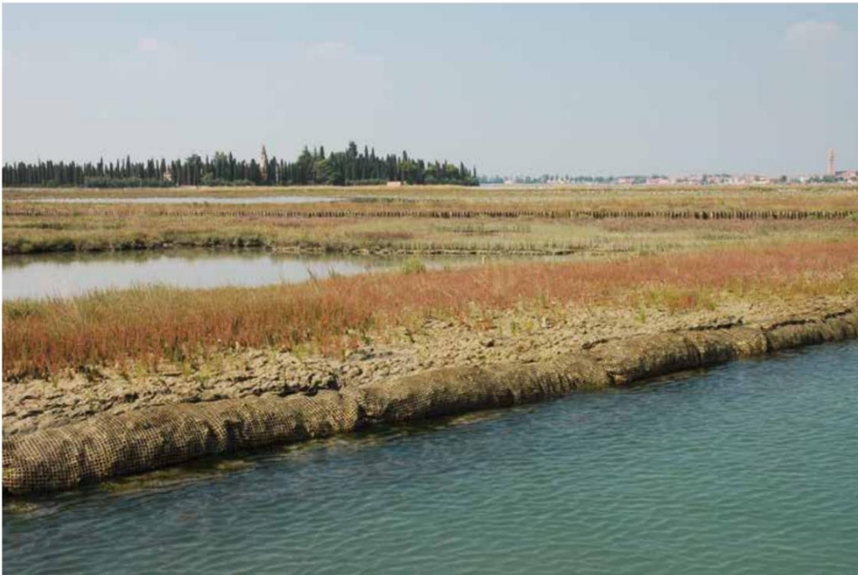
Fig. 10. Gabion "burghe" to protect the edges of artificial and natural salt marshes
