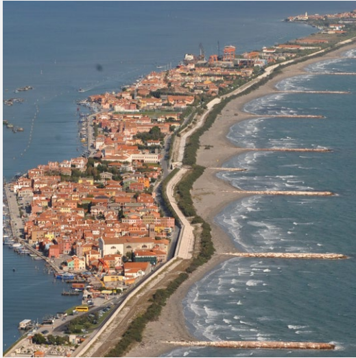
56 km Protected beach nourishment
