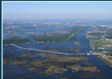
Lake Borgne Surge Barrier
