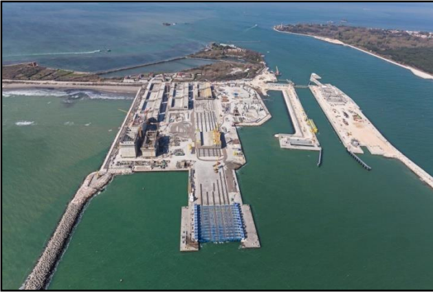
Foto 13 – Prefabrication site of the foundation caissons in Malamocco
