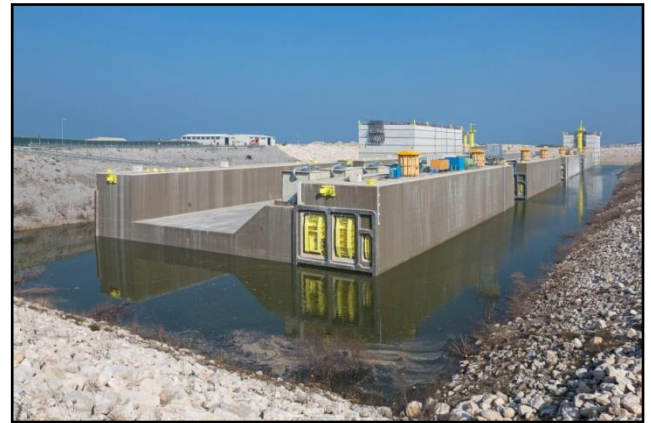
Foto 16 – Complete foundation caissons before being transported to the site while floating
