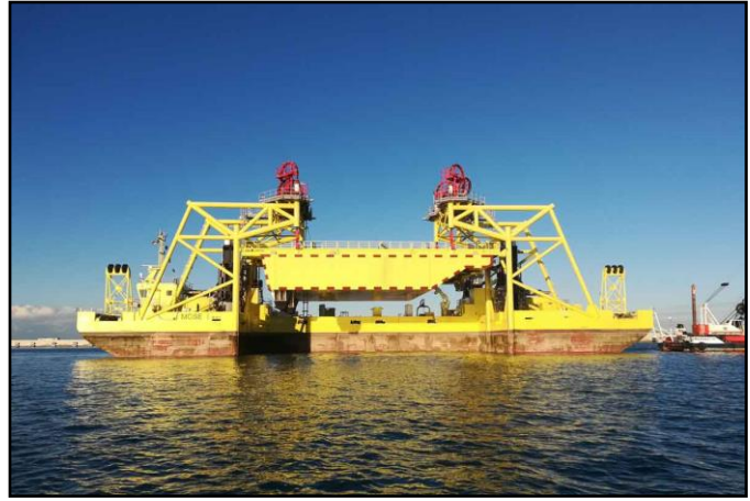
Foto 12 – Jack-ups for transport on site and launching of sluice gates.
