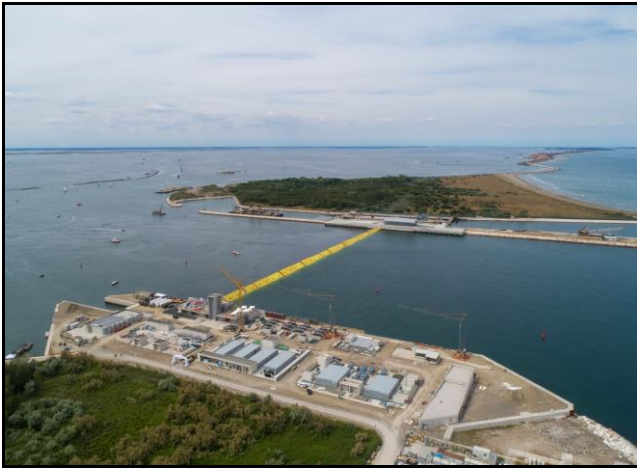
Foto 20 – Mose at Chioggia in operation
