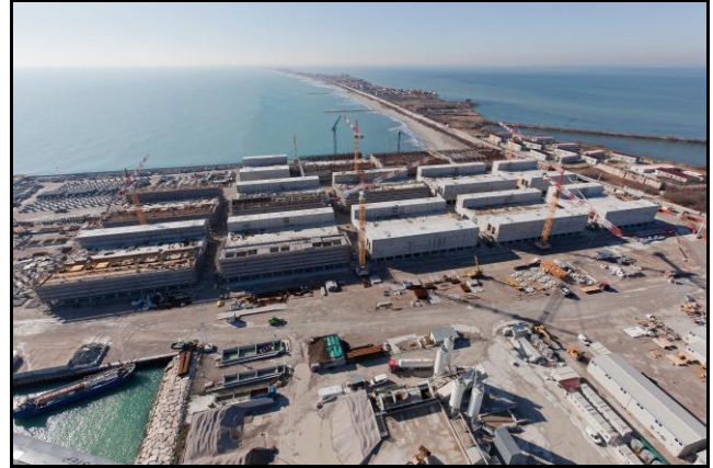
Foto 14 – Containers in the pouring and maturation phase
