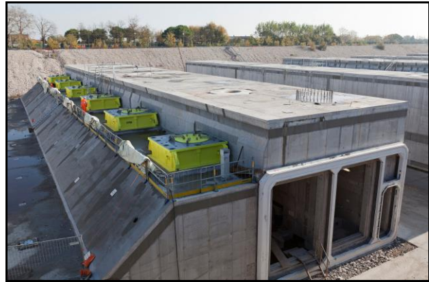
Foto 18 – Foundation box with female elements (yellow).
