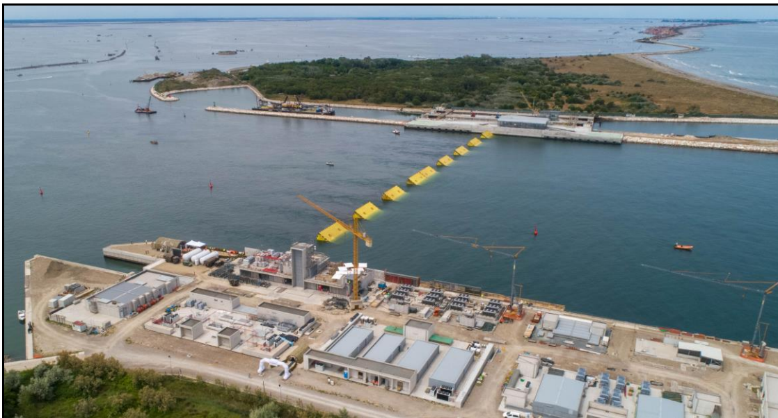
Foto 22 – Partial lifting of the Mose at the mouth of Malamocco
